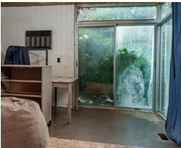
sliding glass door from inside
