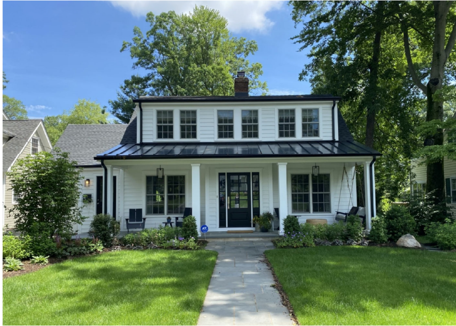
Reference Photo 1: Full-width shed dormer, standing seam metal porch roof, traditional lap siding, white windows, and covered front porch.
