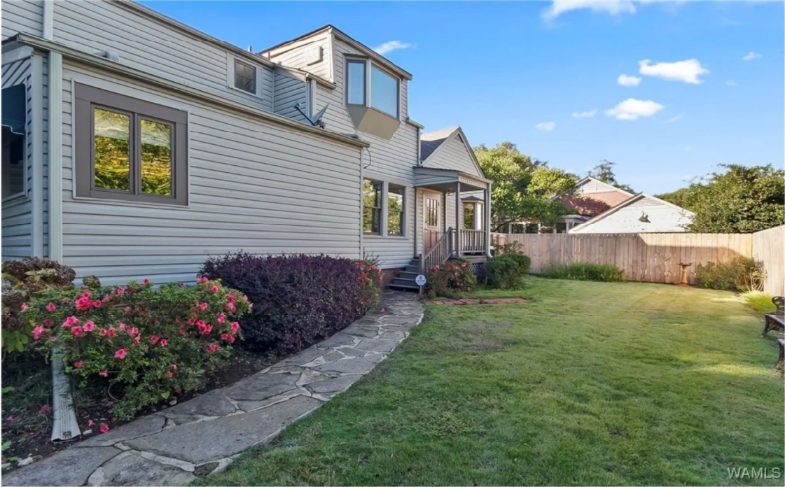
View of the existing rear elevation prior to renovation. Existing dormers limit usable second-floor space and headroom. Proposed improvements include a new shed dormer and a screened rear porch framed with treated lumber and finished with Trex decking materials.
