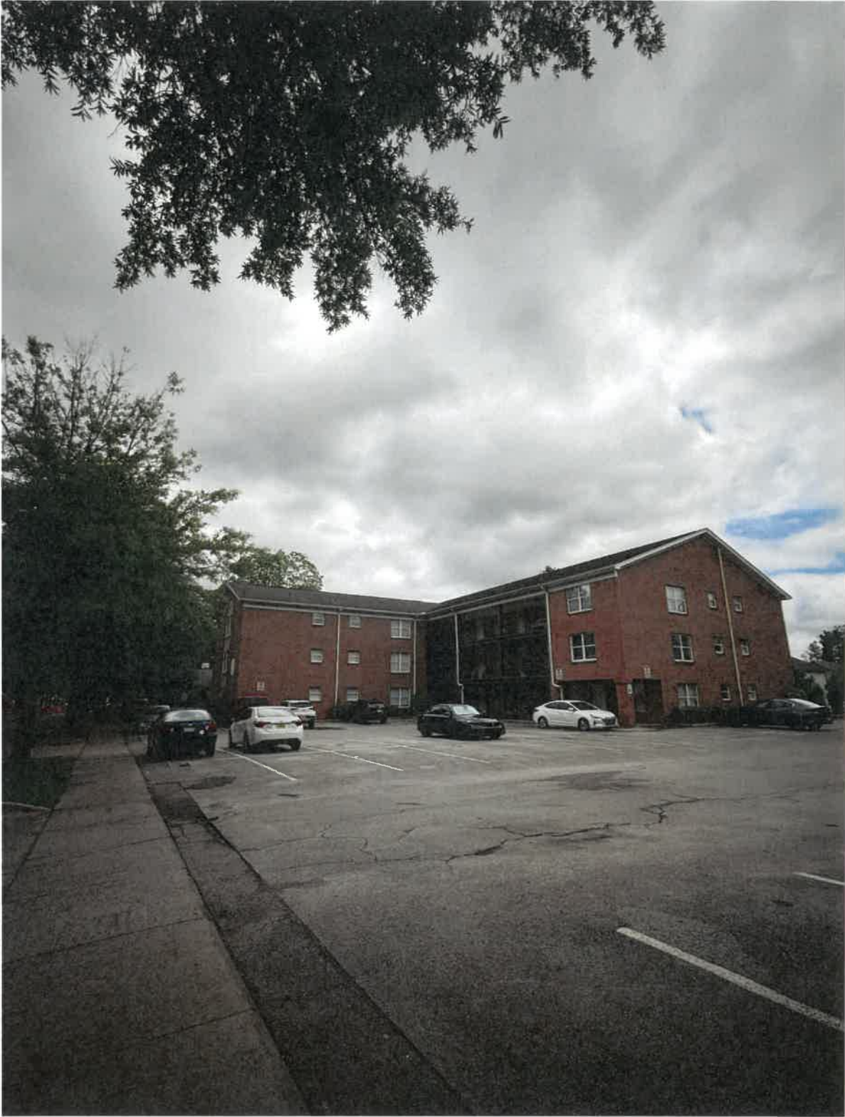
Facing Bryant Drive Apartments from Subject Property
