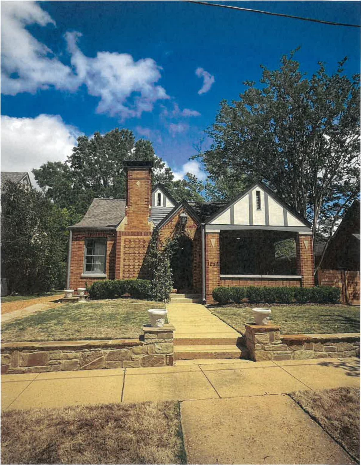
Interior Home in Myrtlewood Heights Subdivision
