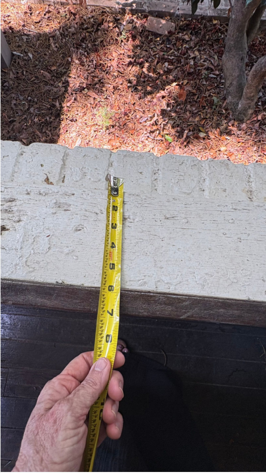
6 x 44 inch window casing (wooden) is already there for large window facing west.
