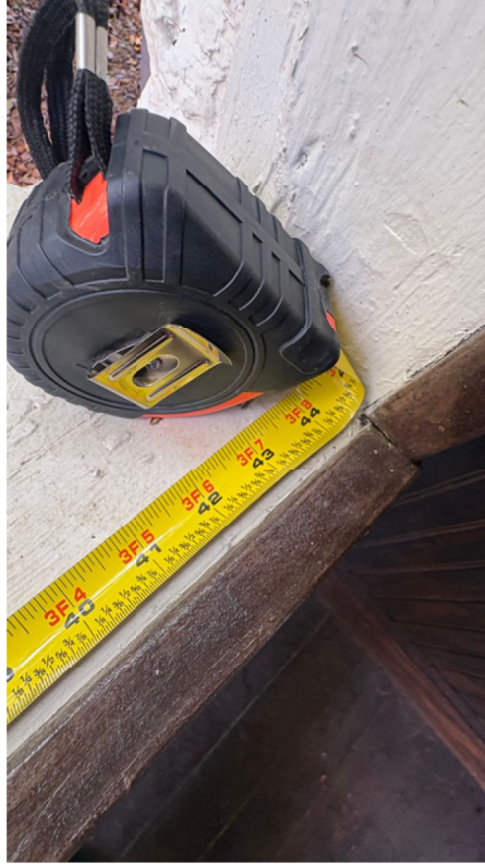
6 x 10 window facing south
