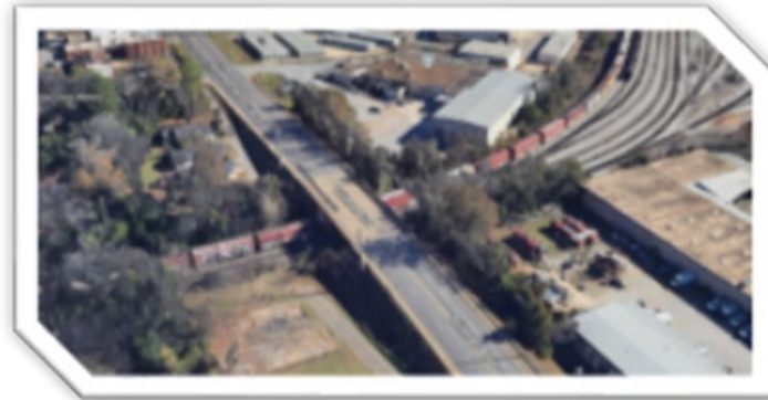
Before: Figure 2. Photo of the current Stillman Boulevard Bridge
