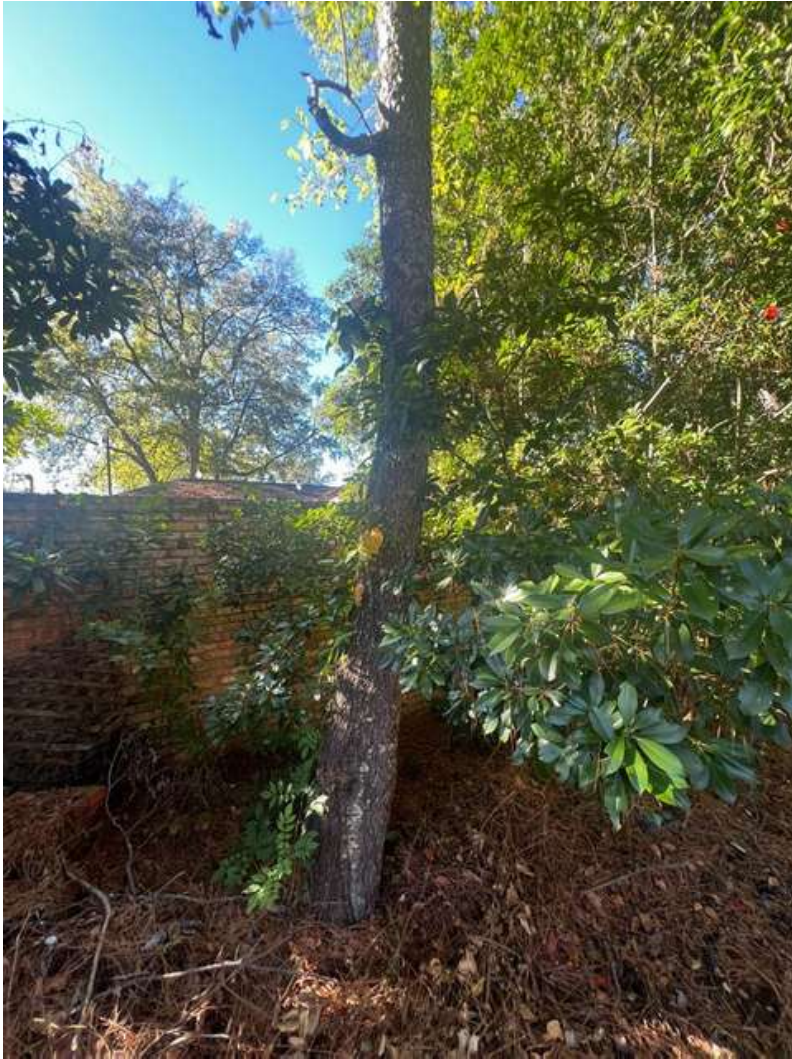
TREE 4 IMPACTING WALL OF 10 PINEHURST GOWING AT AN ANGLE (HERE PICTURED WITH TREE 2 WHICH COULD IMPACT 10 PINEHURST OR SHED AT 19 PINEHURST
