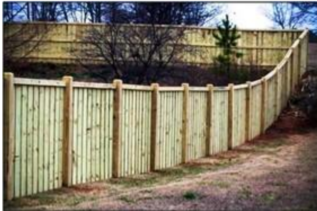
Figure VI-6: Finished Side Facing Exterior
