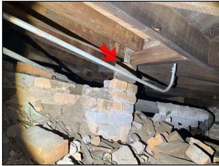
15. Mortar deterioration
