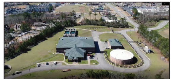
Jerry Plott Water Filtration Plant 2101 New Watermelon Road Tuscaloosa, Alabama 35406 Telephone 205-248-5600
